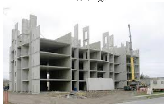
Plate (4) Loaded bearing walls building.
